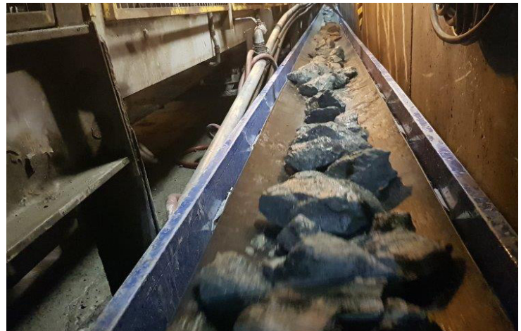
Modulaveyor on-site in an Iron Ore Mine in Tasmania
