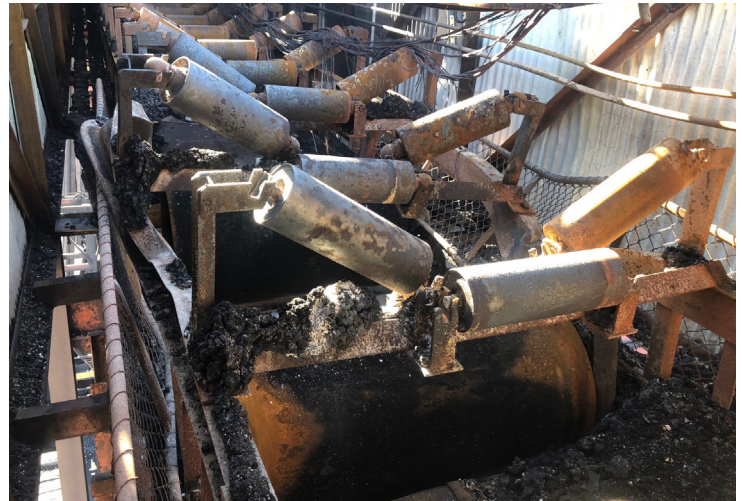
A fire damaged the main conveyor at the Steelworks
